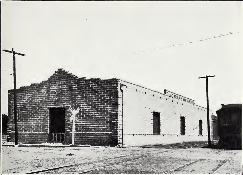
A. ENDURANCE OF WALLS TIED TOGETHER WITH STEEL RODS, LEE BROTHERS' WAREHOUSE, SANTA ROSA.
